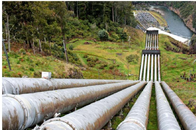
A pumped hydroelectric storage power plant in Tasmania. The plant stores electricity by pumping water uphill when power is abundant. Later, the water flows downhill through turbines, generating electricity during periods of high demand. GETTY IMAGES
